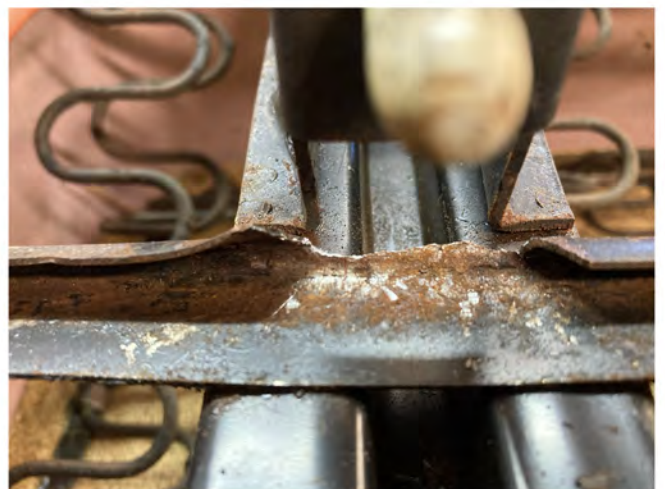
Fig. 4 Remove the center section between the cuts.
